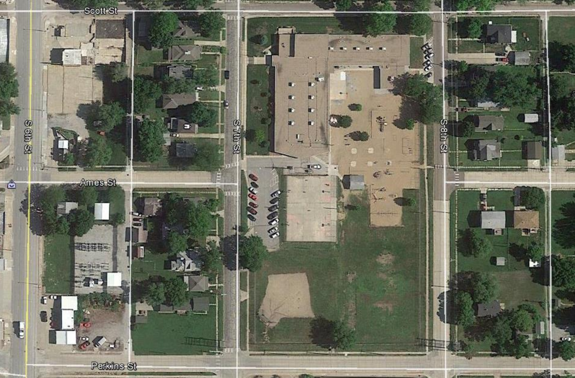
Stoddard Elementary School Site
